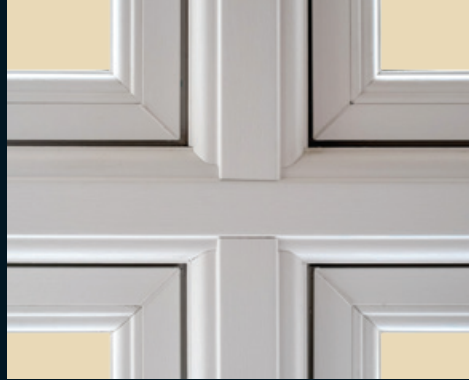
Arrissed joints mimicking traditional timber joinery
